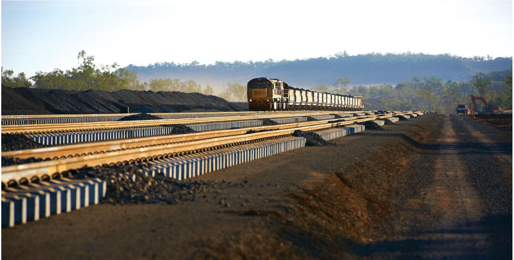
A ballast train completing track work on the Northern Missing Link
