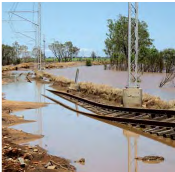
Images above: Rail track washed out from January 2011 floods (left) and repaired (right) at the Comet River on the mainline of the Blackwater System, approximately 40km east of Emerald
