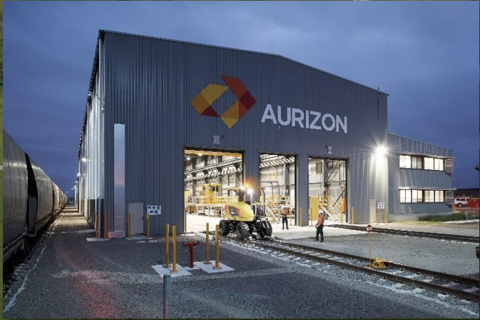
Hexham Train Support Facility, New South Wales
