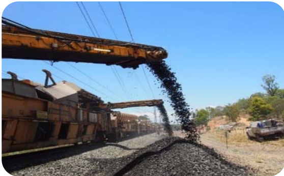
Ballast Undercutting Machine in Operation
