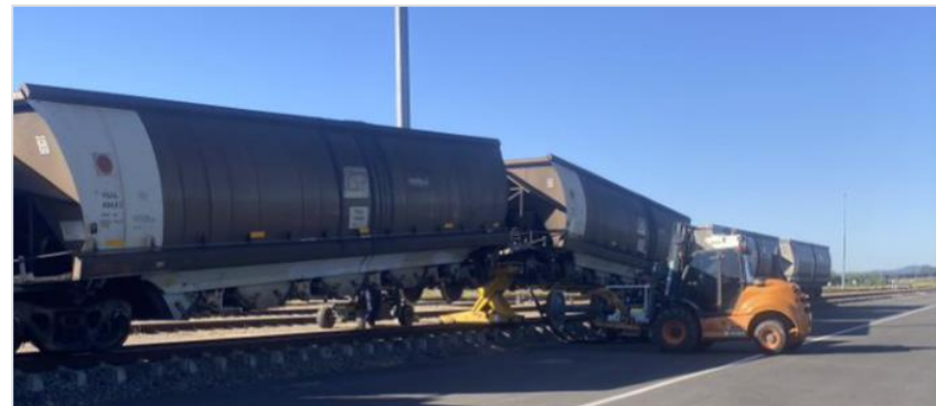
On Train Repair at Jilalan yard
