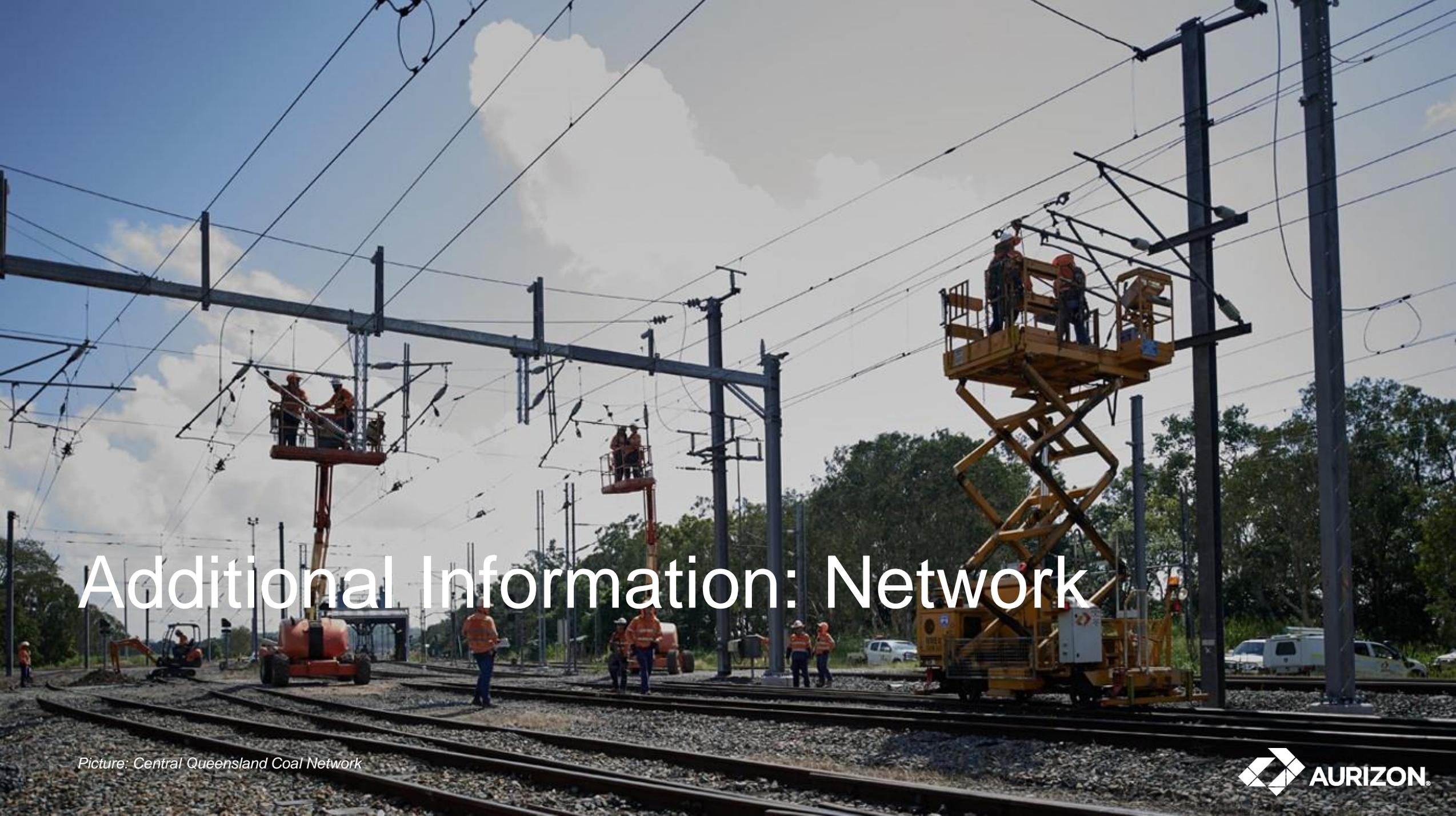
A wide-angle photograph of a railway maintenance site. Several workers in orange safety gear are positioned on yellow scissor lifts, working on the overhead power lines. The scene is set against a blue sky with scattered white clouds. In the foreground, there are multiple parallel railway tracks on a gravel bed. The background shows some greenery and a few parked vehicles.
