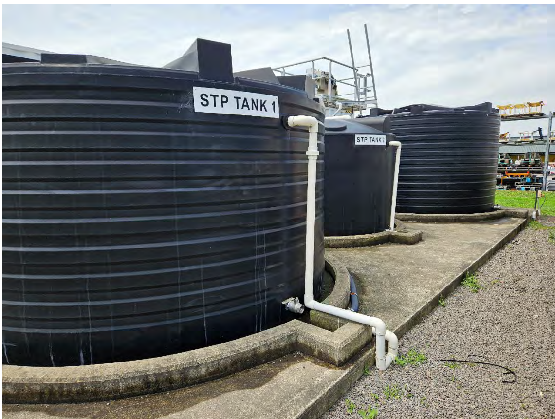
Photo 11. On-site sewage treatment plant - tanks
