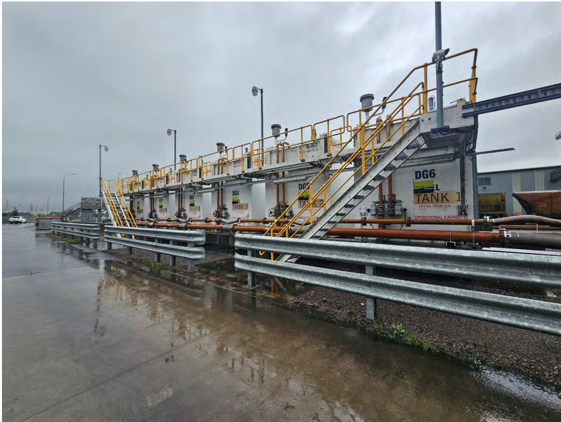
Photo 20. Provisioning facility, ASTs. Braided sections of pipe visible.
