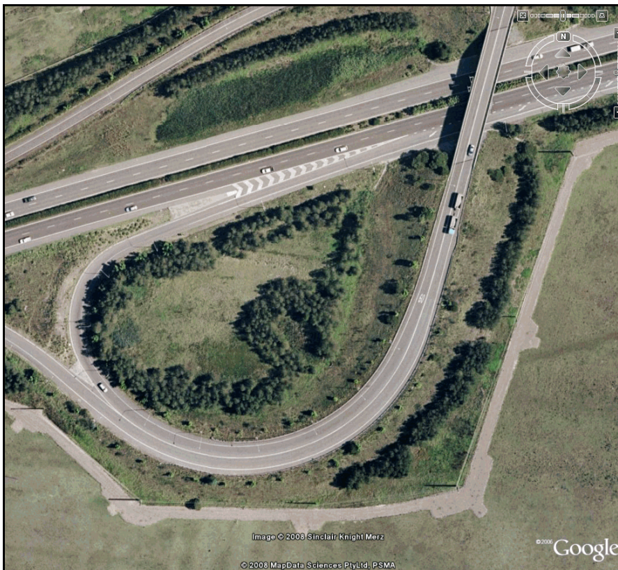
Figure 1: Southern Abutment of Tarro Interchange
