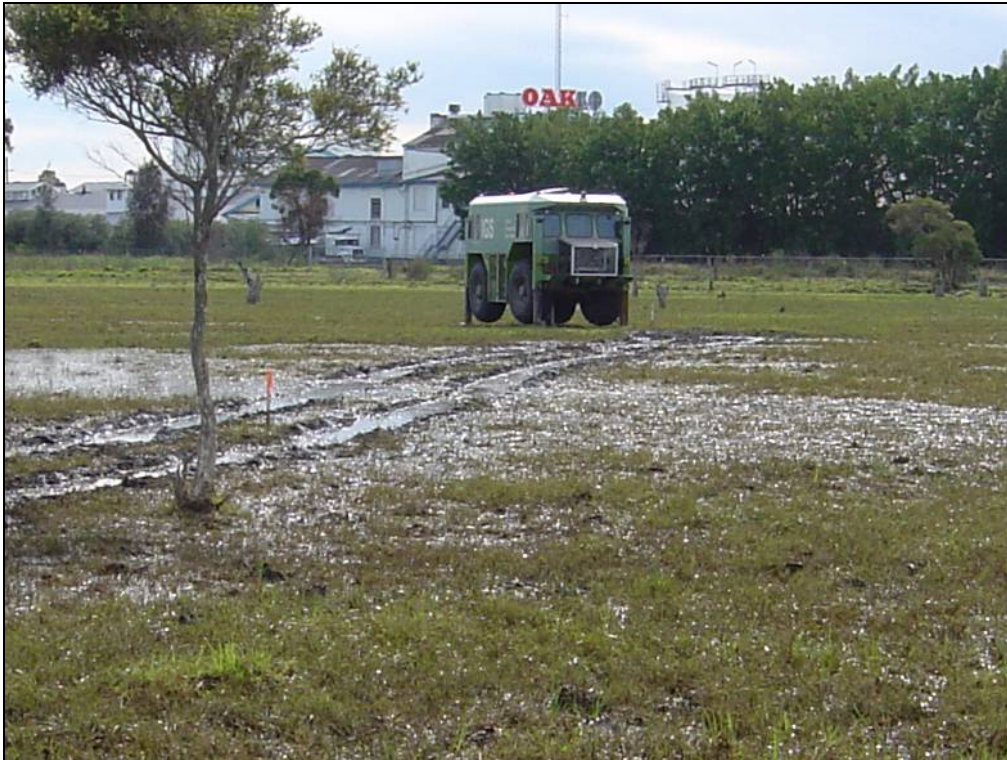
Figure 9: CPTu testing within low lying parts of the site using “all terrain” rig (2007)
