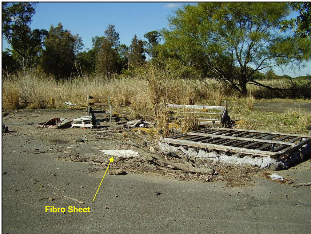
Figure 4: Scattered filling over a paved area in the central part of the site
