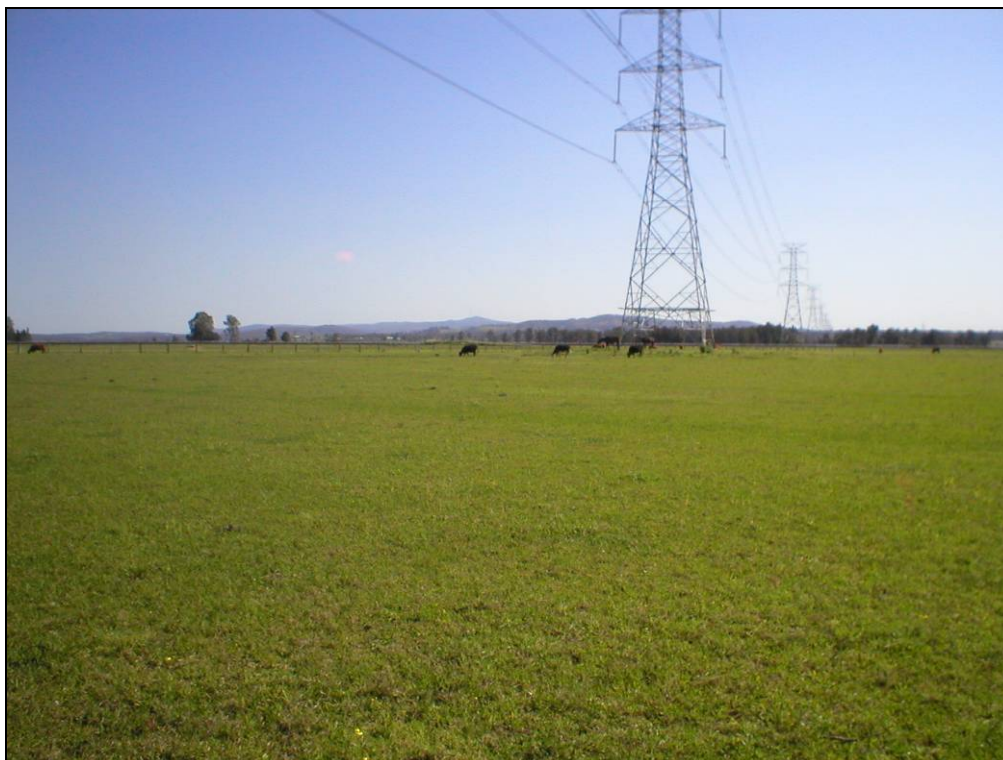
Figure 8: Western part of the site
