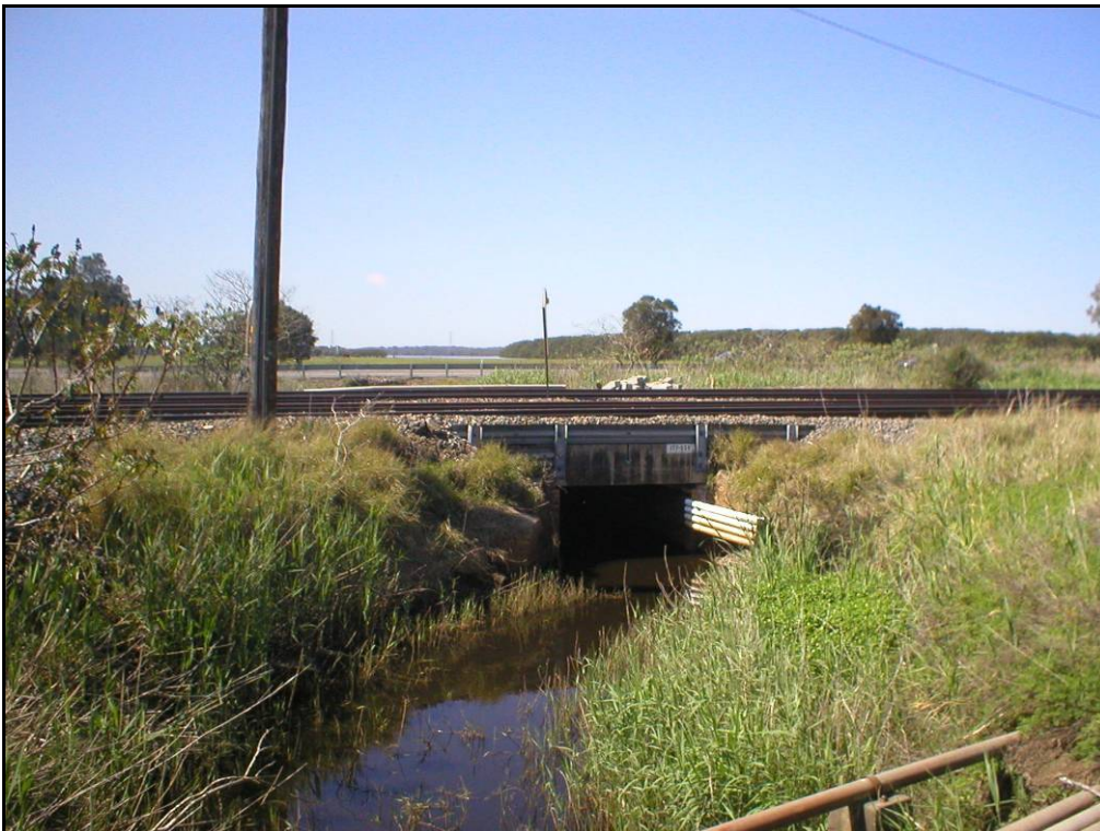
Figure 7: Culvert beneath existing track at Ch 177.060 km
