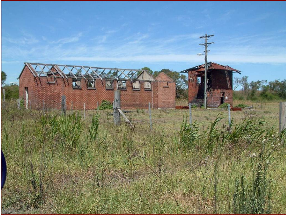
Photograph 7: Former bathhouse and control box/lunchroom
