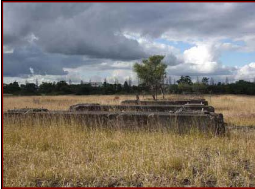
Photograph 18: Conveyor belt support footings.
