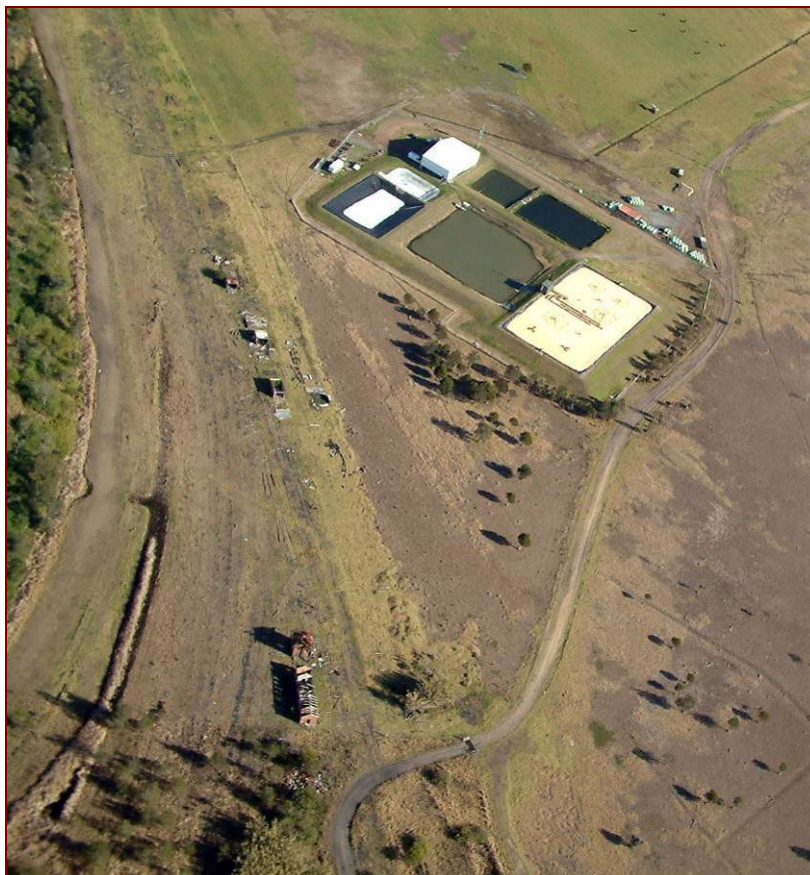
Photograph 8: Brancourts' waste water treatment facility
