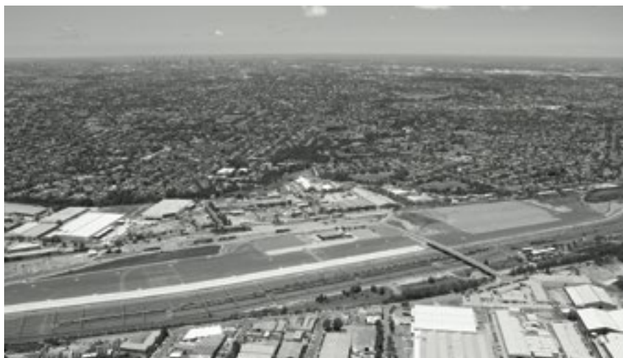
The new Aurizon Enfield depot in Western Sydney.
