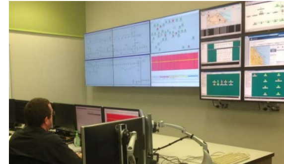
Fault Control Centre
