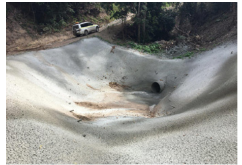
Photo: Black Mountain Debris Protection Barrier, May 2018. Black Mountain Shotcrete Inlet, May 2018, Black Mountain Stabilisation Works.
